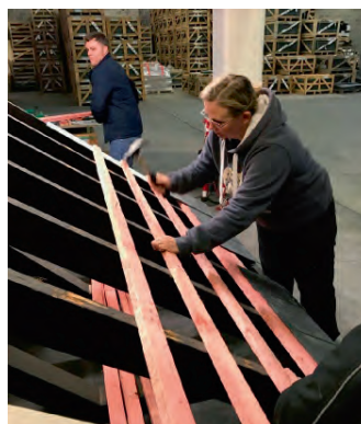
Sam learning how to lay roof slates
